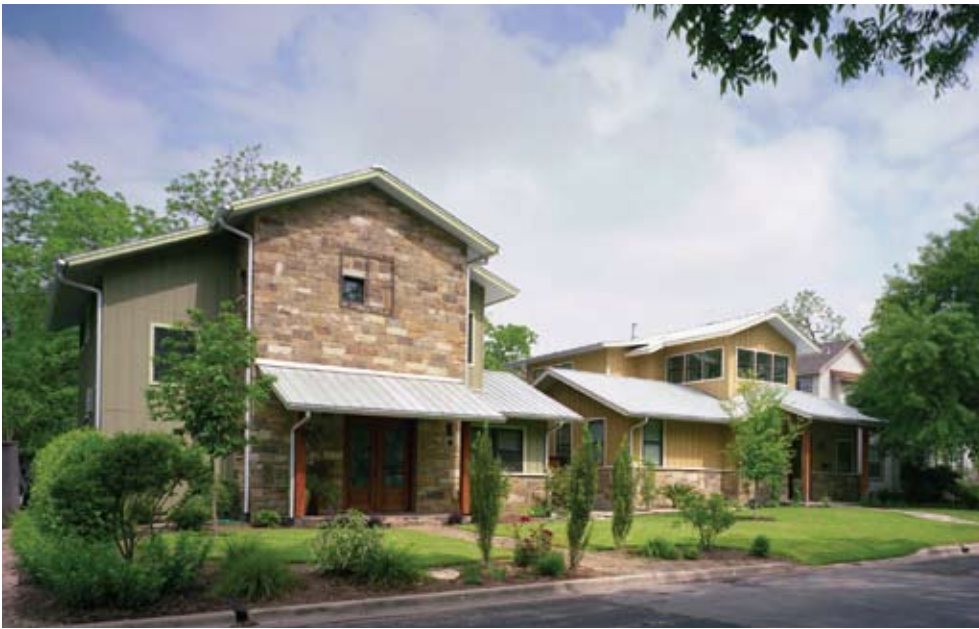
Left to Right: Galvalume standing seam reflective metal roofs on two new green-built homes. Spray polyurethane foam insulation in Jay's attic.
